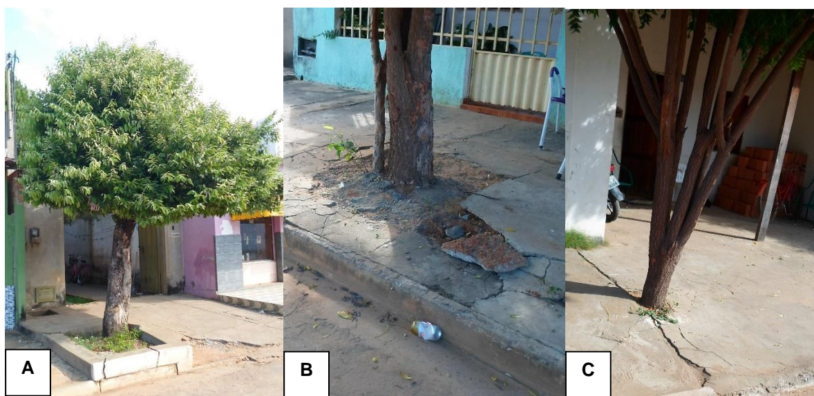
Figura 3. Raízes afetando as calçadas. (A) Licania tomentosa . (B e C) Azadirachta indica Figure 3. Roots affecting the sidewalks. (A) Licania tomentosa . (B and C) Azadirachta indica
