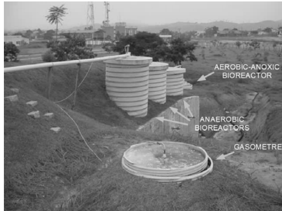
Figure 1. Small wastewater treatment station at UNESP (back view).
