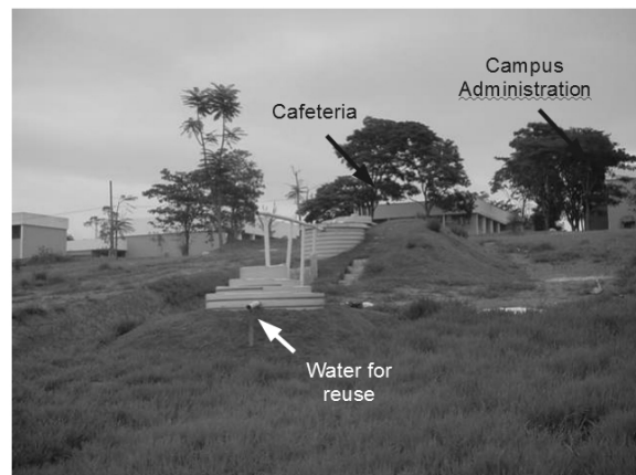
Figure 2. Small wastewater treatment station at UNESP (front view).
