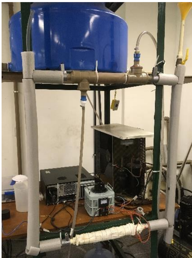
Figure 1: Passive Cooling System built for the project.
