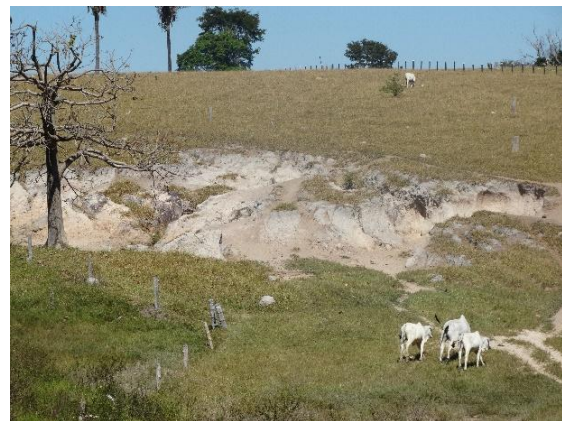
Figure 6 - Erosive processes in areas of Figueirópolis'Oeste– MT. Source: LabGeoUnemat (2017).
