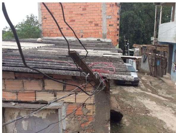
FIGURE 6 – Informal electrical connections in Vila Nova Esperança. SOURCE: the author.
