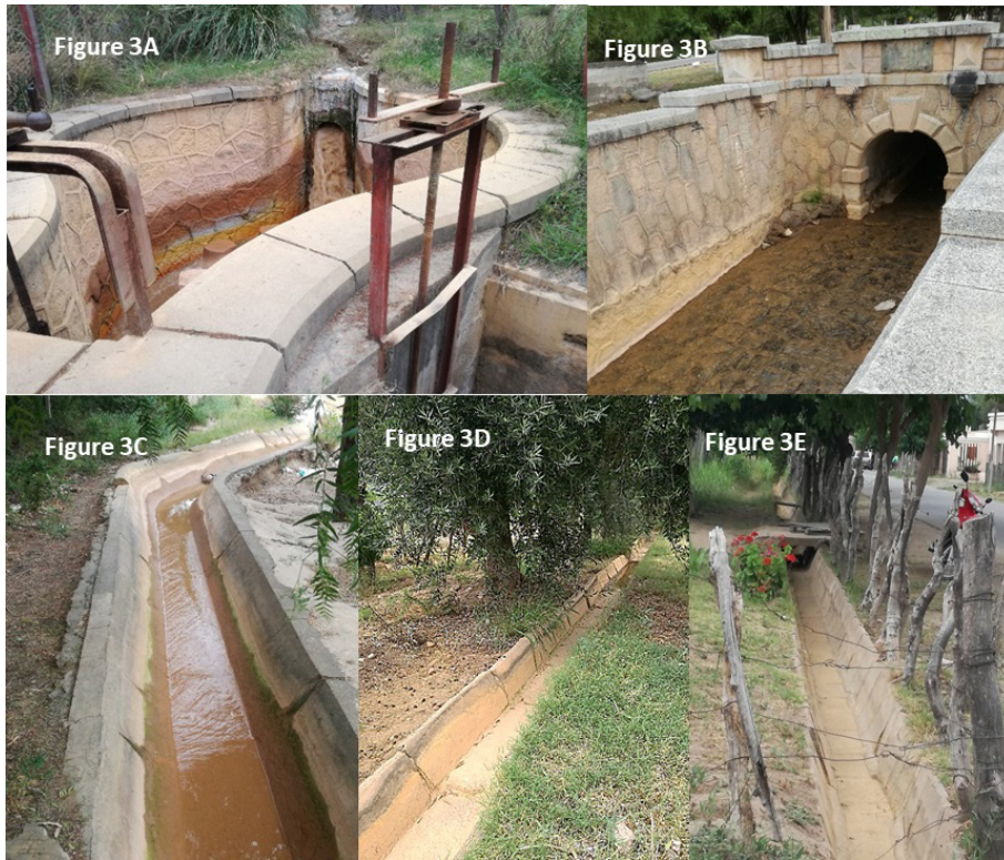
FIGURE 3— Channel matrix in Santa Florentina and network of small channels that irrigate agricultural lands in the District of Malligasta, Antinaco - Los Colorados valley, Argentina.
