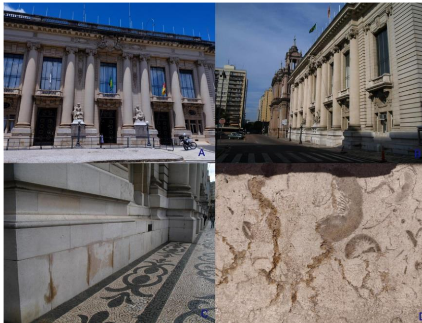
Figure 1. Details of Palácio Piratini. A) Entrance of Palácio Piratini; B) Side view detail; C) Sidewalk with quartz and diabase mosaic; D) Detail with marine fossils.
