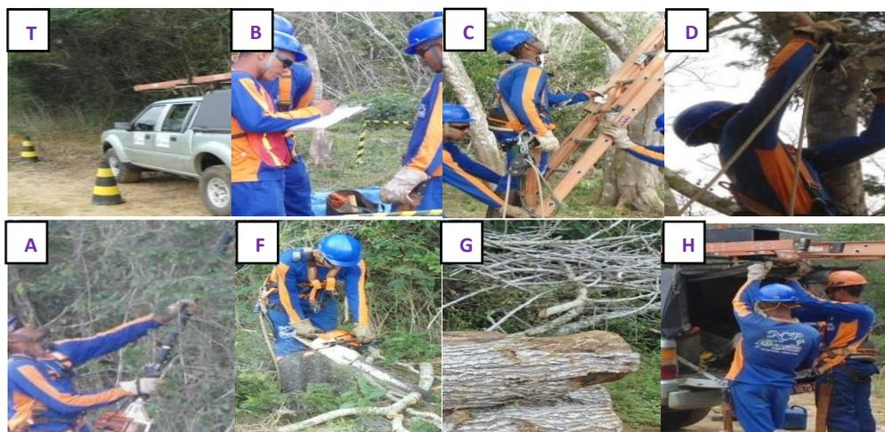
Figure 1. Operational process of pruning trees conflicting with power lines. A - Signaling; B – Completion of the Preliminary Risk Analysis (PRA); C - Ladder position; D - Height work kit positioning; E - Pole saw; F- Process operation with chainsaw; G – Cut logs; H - Material storage.
