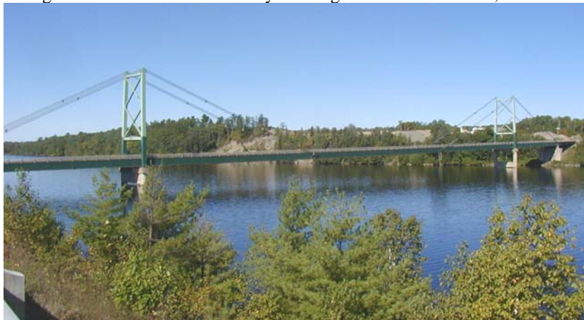
Figure 8 - Hawkshaw Cable-stayed Bridge in New Brunswick, Canada.
